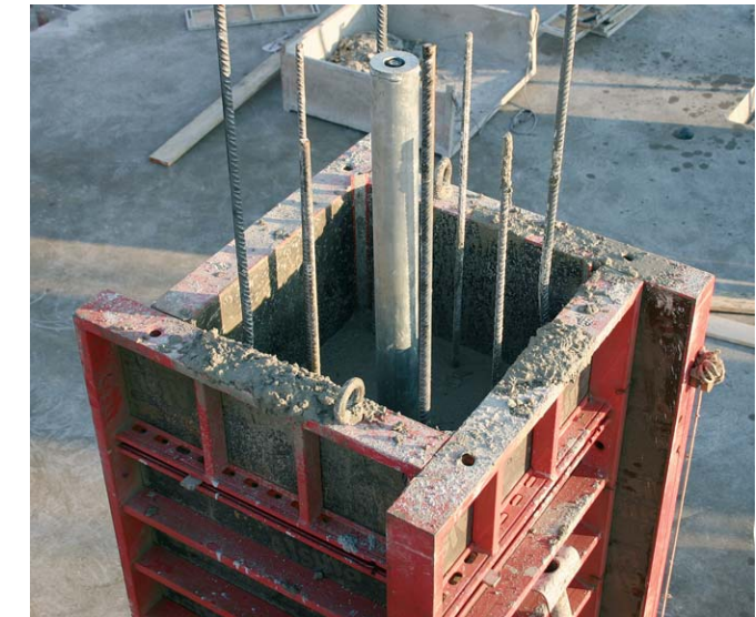
*Studies by Accredited Bodies, available to our customers on request, indicate that a column with the tube cast-in, does not impair its strength.
